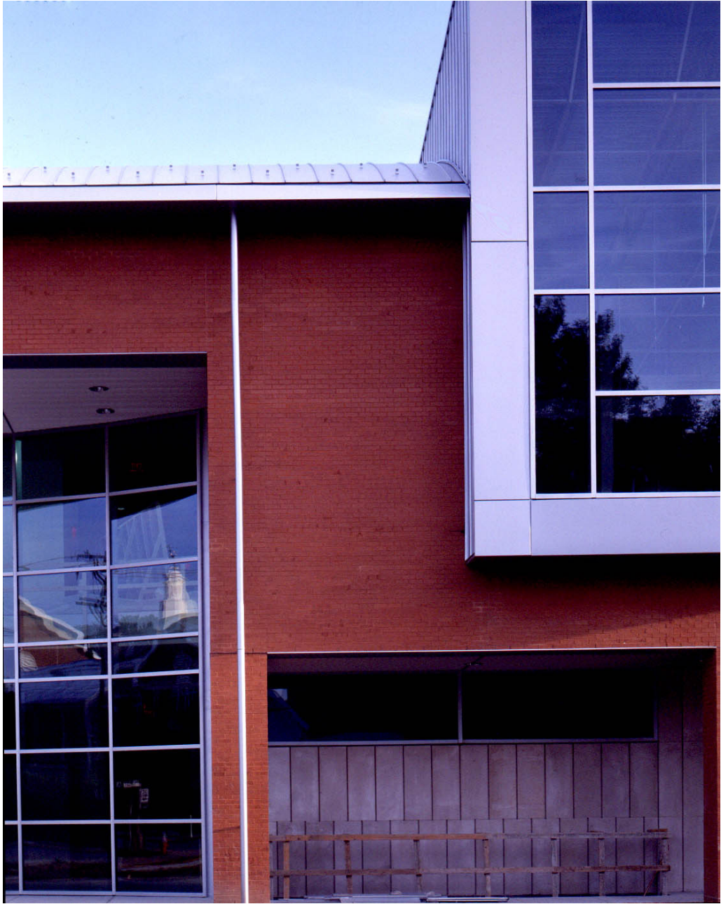
Detail of main entrance colonnade
