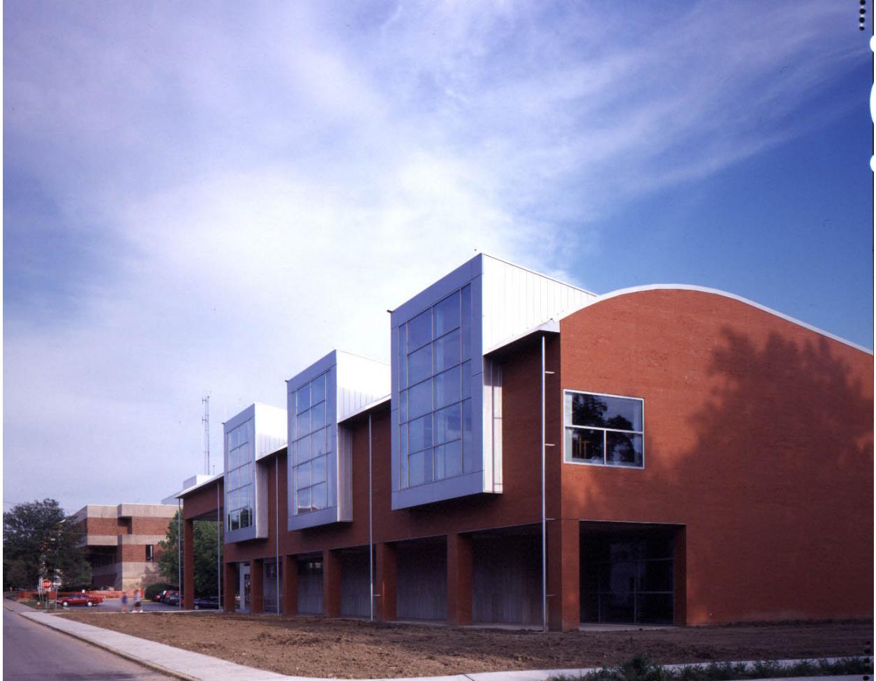
View of northwest façade at the intersection of Hanna and Jackson streets
