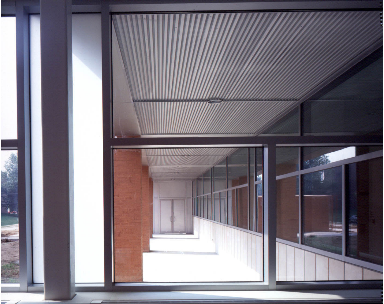
View of east colonnade and interior courtyard
