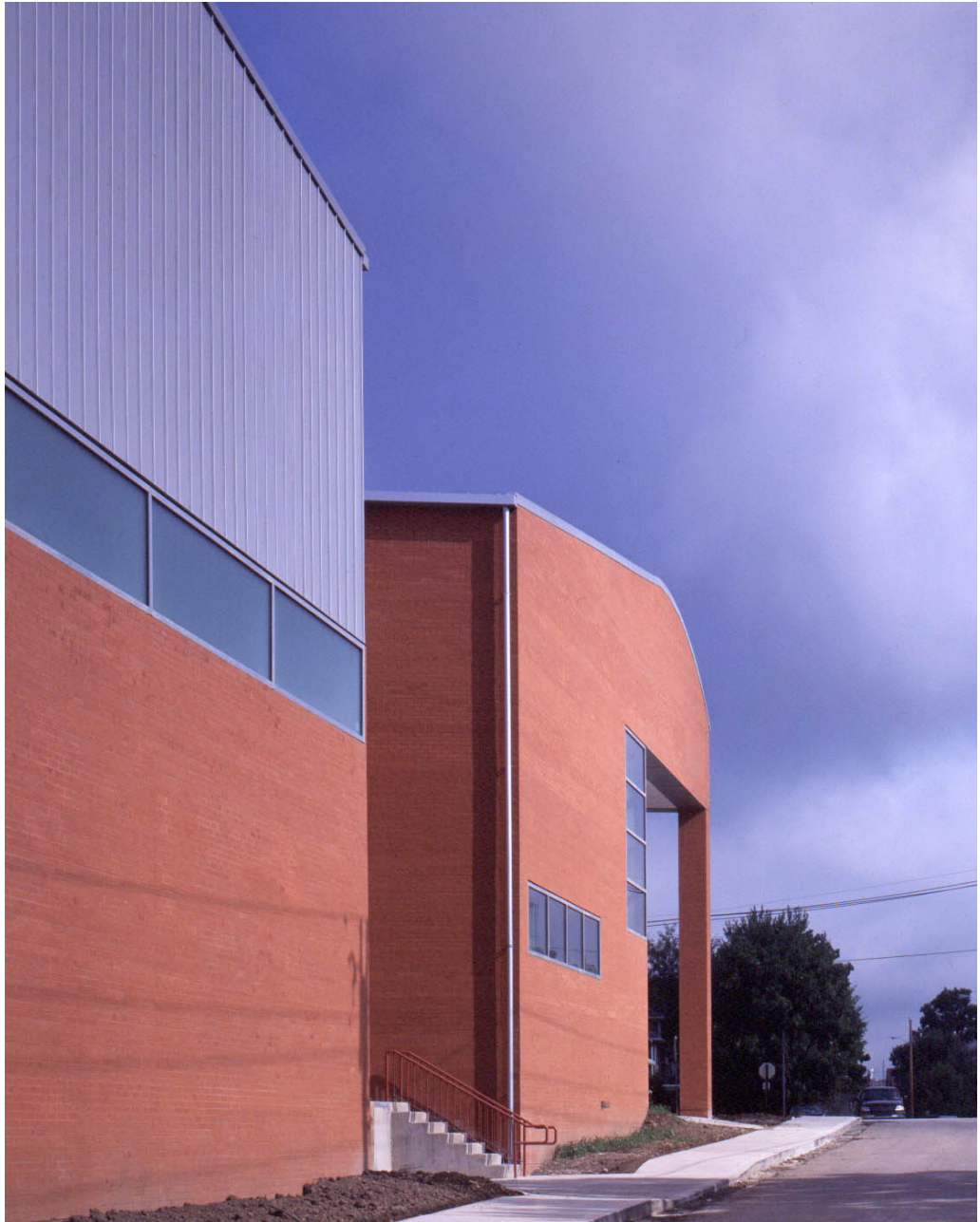
East façade viewed from Indiana Street
