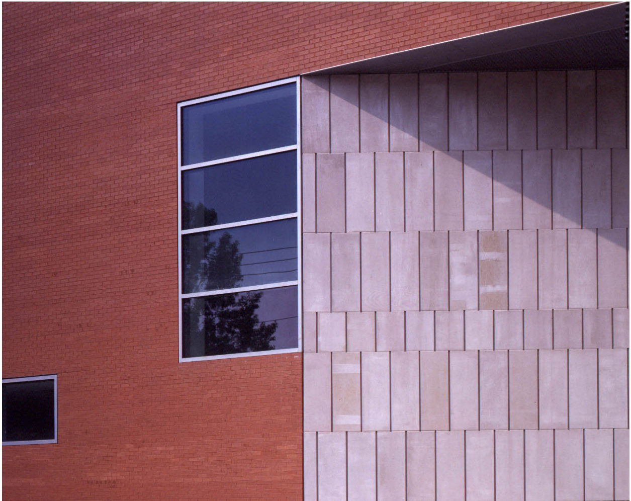
Detail of east façade
