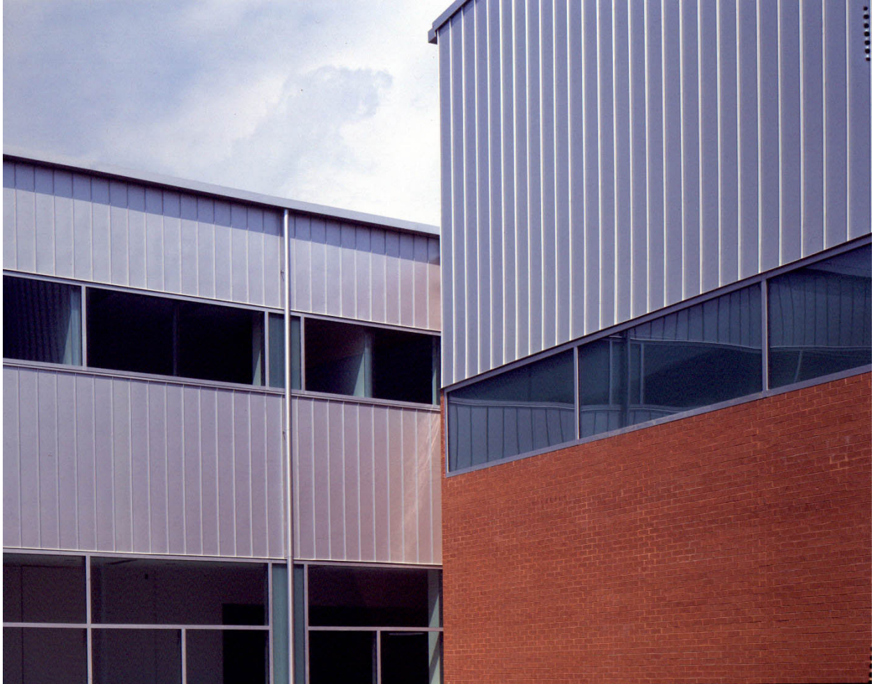
Close-up detail of main gallery volume at interior courtyard.
