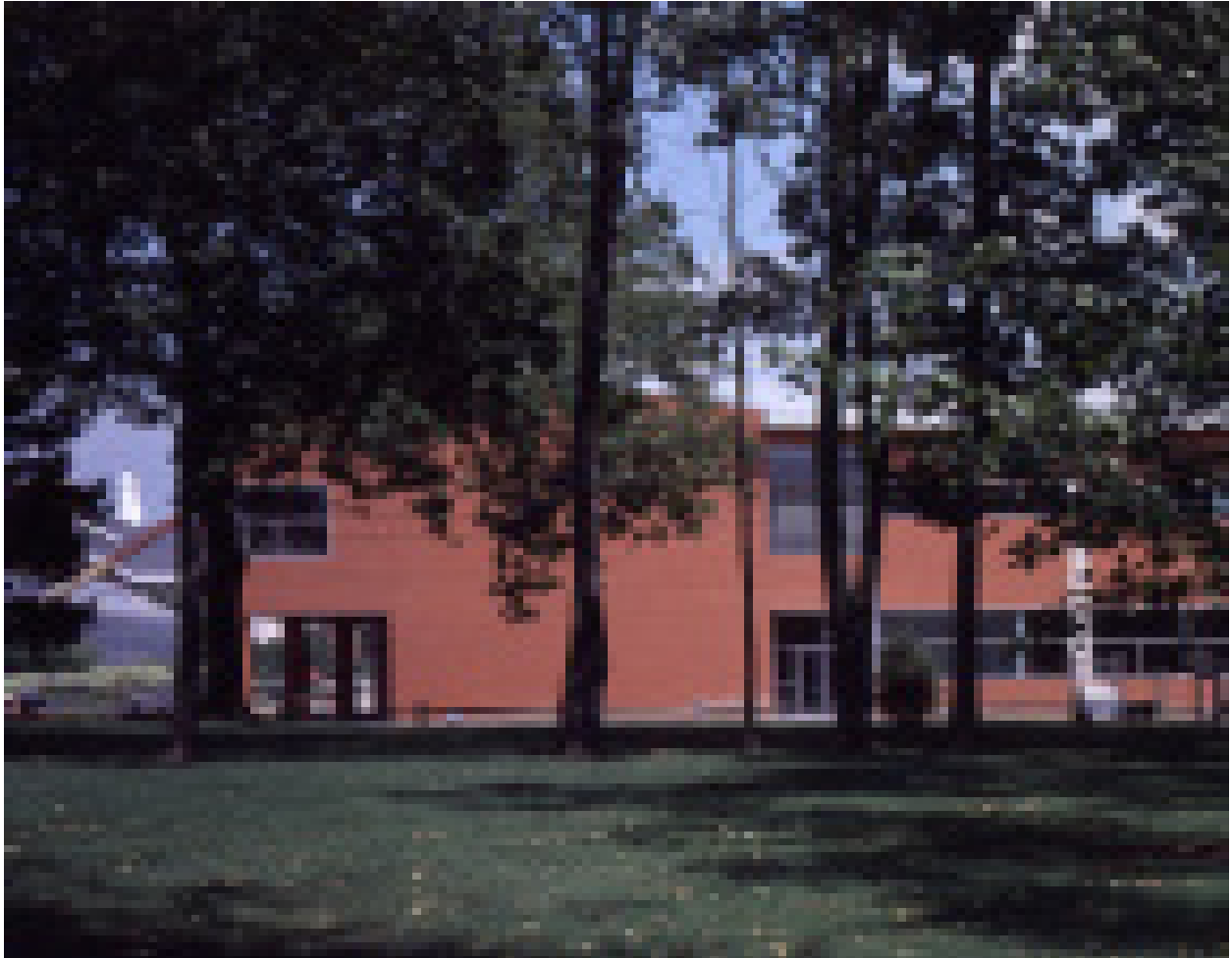
View of west façade from adjacent park
